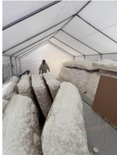
Figure 5: EnviroSeal OC Platinum Application with Active Ventilation
