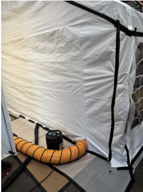
Figure 5: EnviroSeal OC Platinum Application with Active Ventilation
